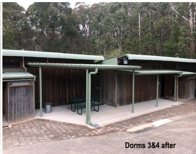
Two dilapidated dorm verandahs were replaced, and an additional verandah at dorms 3&4 was constructed. The new decking material is floating concrete for fire safety reasons. Paving and storm water drainage is also improved.
