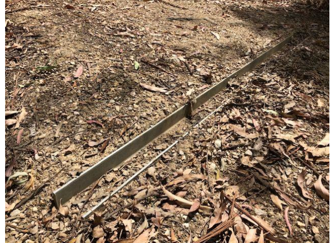
Erosion control trials and track maintenance. Steel 'C' channel is an effective and easy to manage solution to a long standing problem.
