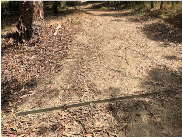
Erosion control trials and track maintenance. Steel 'C' channel is an effective and easy to manage solution to a long standing problem.
