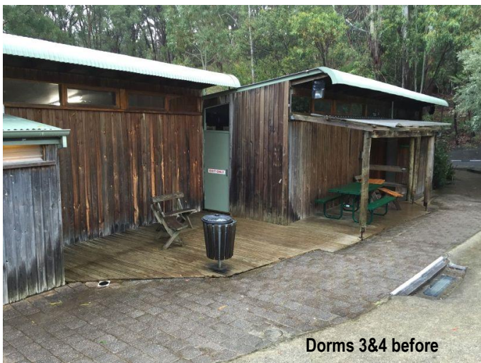
Two dilapidated dorm verandahs were replaced, and an additional verandah at dorms 3&4 was constructed. The new decking material is floating concrete for fire safety reasons. Paving and storm water drainage is also improved.
