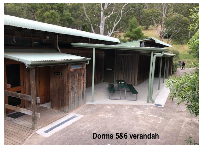
Two dilapidated dorm verandahs were replaced, and an additional verandah at dorms 3&4 was constructed. The new decking material is floating concrete for fire safety reasons. Paving and storm water drainage is also improved.
