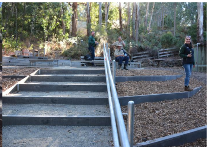
The tired looking campfire area received some TLC in January. It now has wide concrete steps, adjacent terracing with low plants, and downlights for nighttime accessibility.
