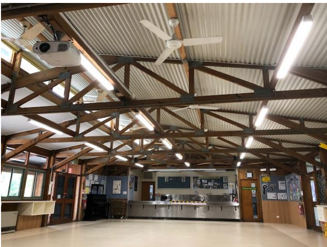
Dining room fluoro lights were replaced with energy saving LED tubes.
