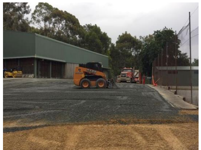
Driveway and carpark was relevelled and resurfaced.
