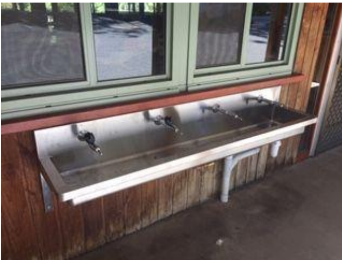
A stainless steel drinking and bottle filling trough replaced an old water bubbler. Less leaks and puddles next the dining room entry.
