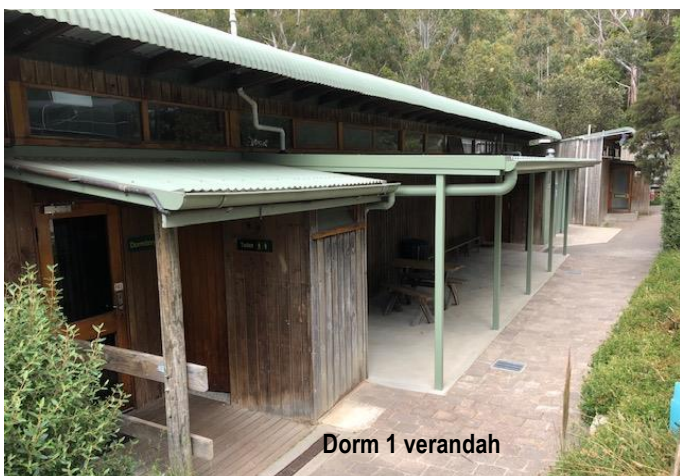
Two dilapidated dorm verandahs were replaced, and an additional verandah at dorms 3&4 was constructed. The new decking material is floating concrete for fire safety reasons. Paving and storm water drainage is also improved.
