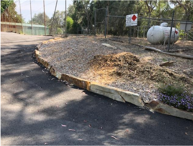
Stone edging wall and line marking in the newly laid bitumen carpark and driveway.
