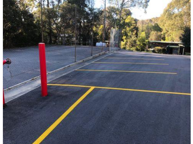
Stone edging wall and line marking in the newly laid bitumen carpark and driveway.
