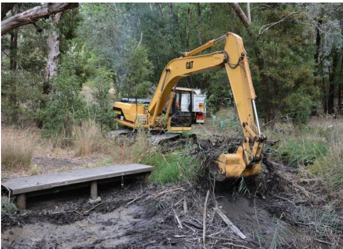
After an unusually dry autumn, it was a good opportunity to dredge pond 3, removing 15 years' worth of silt and sedimentation. A subsequent new timber deck, rock edging and revegetation has rejuvenated this important teaching space.
